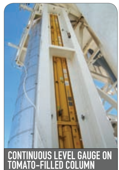
Figure 5. During a 100-day processing season, the gamma level gauge remained constant.
