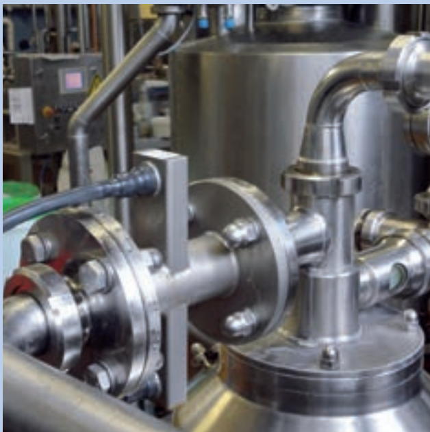
Water-content measurement in a dairy plant – LB 566 with flow cell
