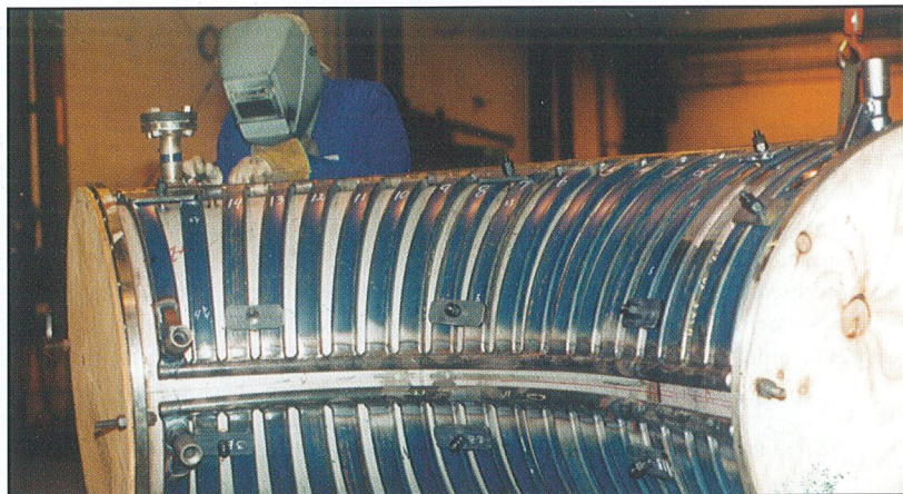
To help prevent plating in the waste gas header, a producer of a common anhydrous material installed new bolt-on heat trace elements to keep the header's wall at a uniform temperature.
