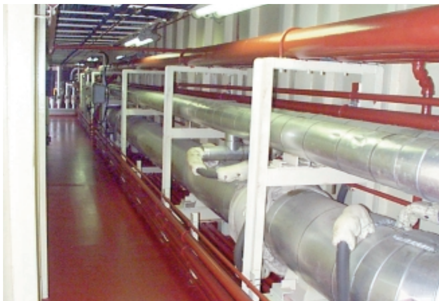
Fig. 4: Bolt-on thermal maintenance systems have operated trouble-free on the Sulphur Enterprise since the ship's launch in 1994.
