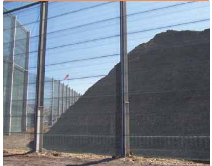
Figure 6. DustTamer can also be used as a stand-alone wind fence system, as shown here, to reduce air movement across a material stockpile.
