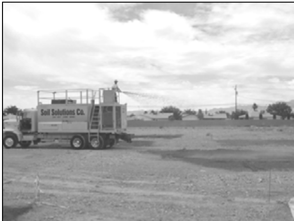
Figure 2-4: Topical application of a dust suppressant using a spray gun.
