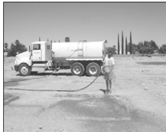
Figure 2-2: Topical application of a dust suppressant using a spray hose.
